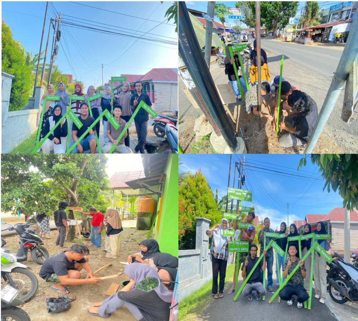
Figure 1. Documentation of the Construction and Installation of Road Crossings
